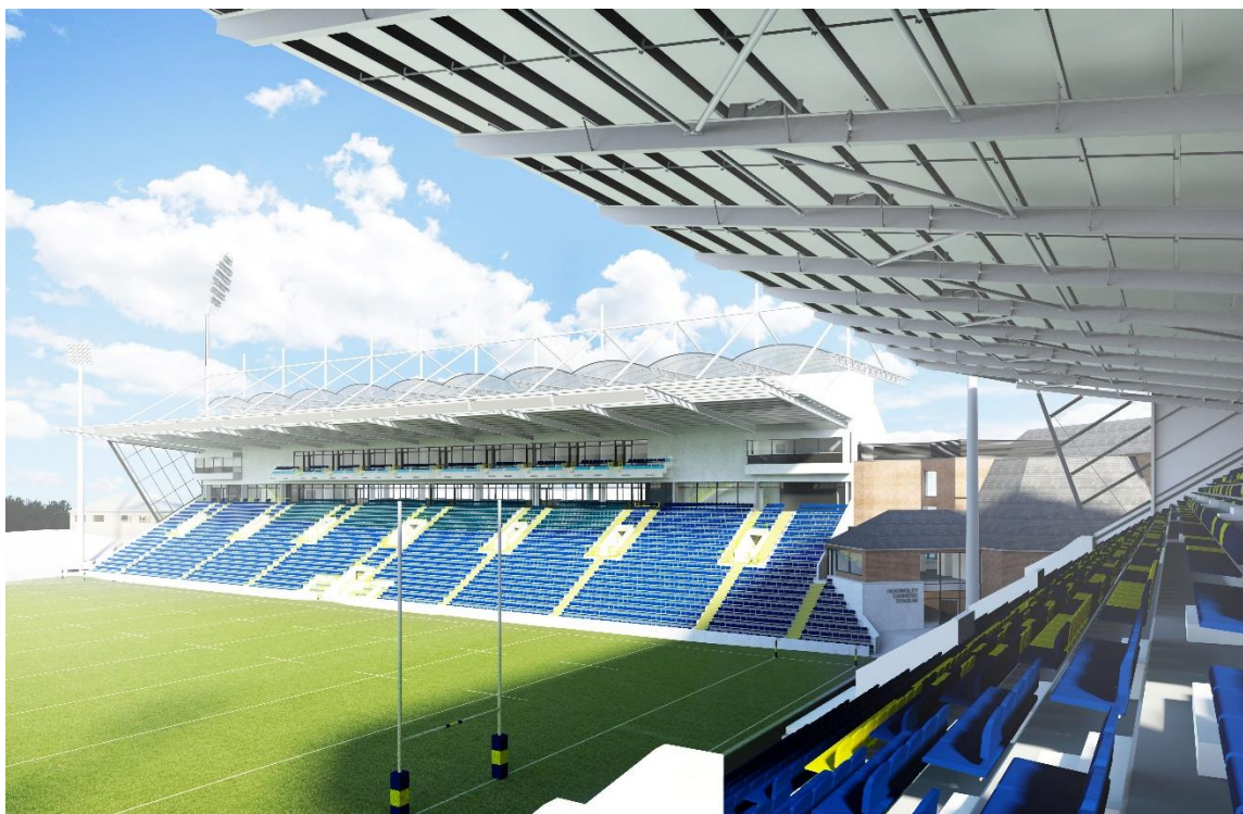
Figure 2.4: Rugby Stadium double facing North South Stand
